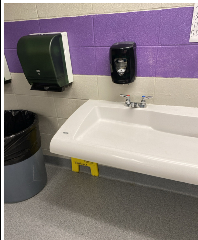
2/8/2024 - 304-43 - Primary School - Daycare-Left
