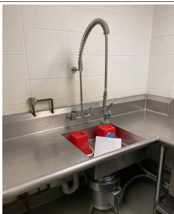
2/8/2024 - 304-56 - Primary School - Kitchen- West Sink
