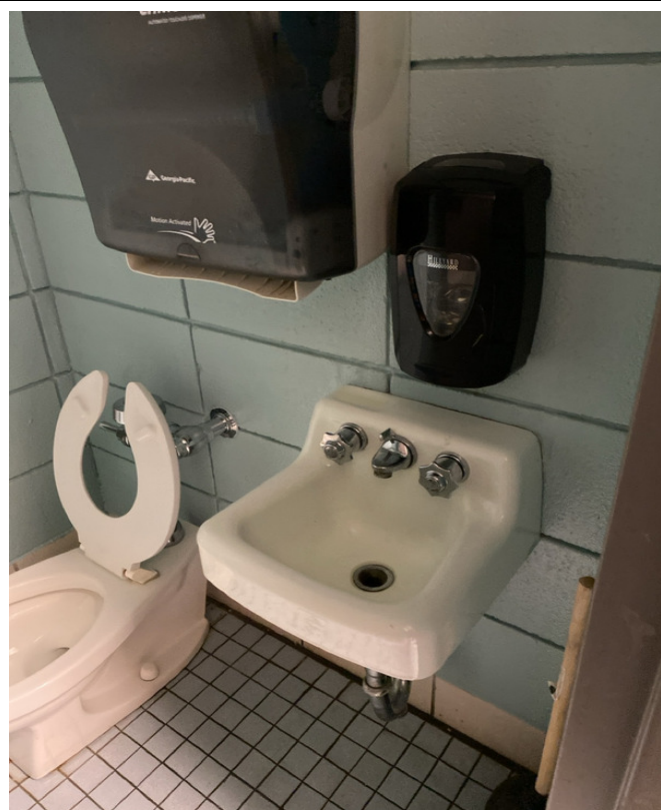
2/8/2024 - 304-48 - Primary School - Room 100- Left Restroom
