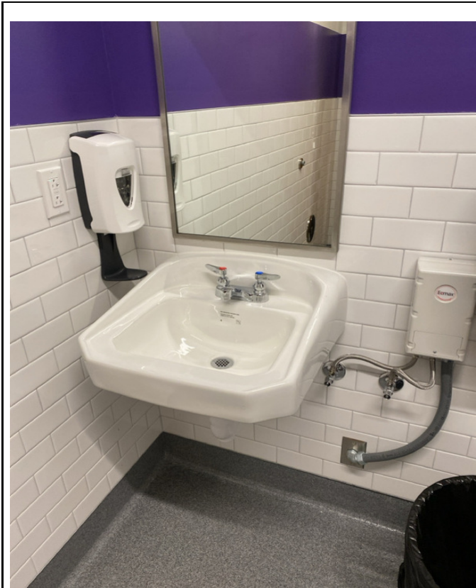
2/7/2024 - 304-13 - Primary School - Library- Restroom
