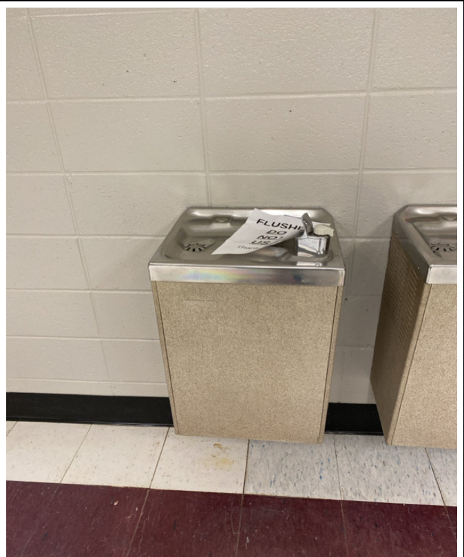
2/7/2024 - 304-24 - Primary School - Outside Room 111-Left
