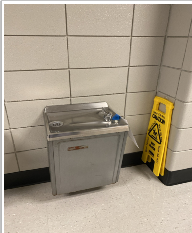
2/7/2024 - 304-9 - Primary School - West Hall by Office-Right
