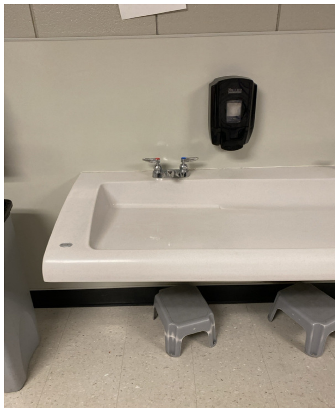
2/7/2024 - 304-5 - Primary School - West Hall by Office-Fourth from Left
