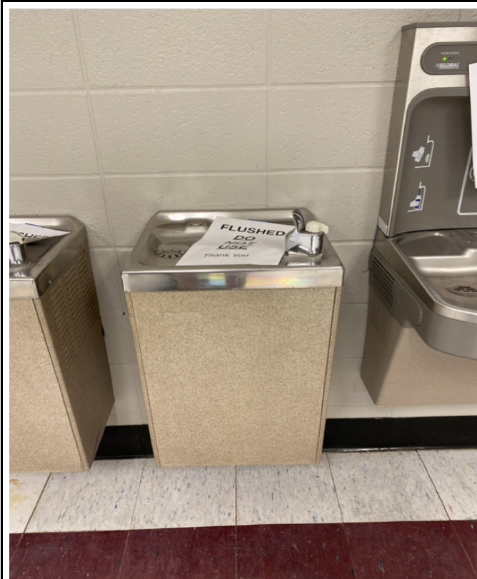
2/7/2024 - 304-25 - Primary School - Outside Room 111-Middle
