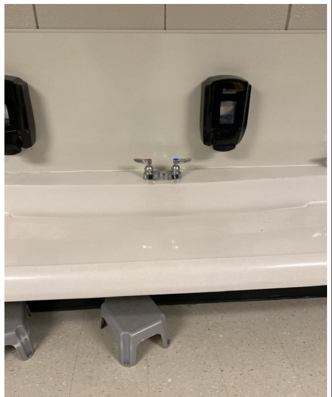
2/7/2024 - 304-6 - Primary School - West Hall by Office-Fifth from Left
