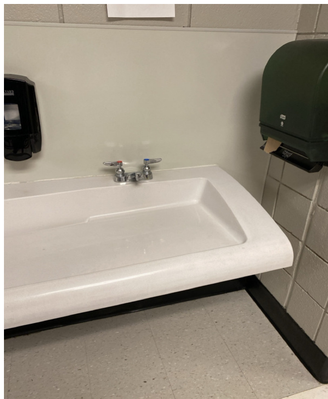
2/7/2024 - 304-19 - Primary School - East Hall by Office-Sixth from Left
