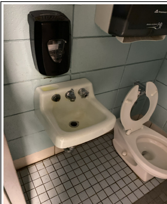
2/8/2024 - 304-49 - Primary School - Room 100- Right Restroom
