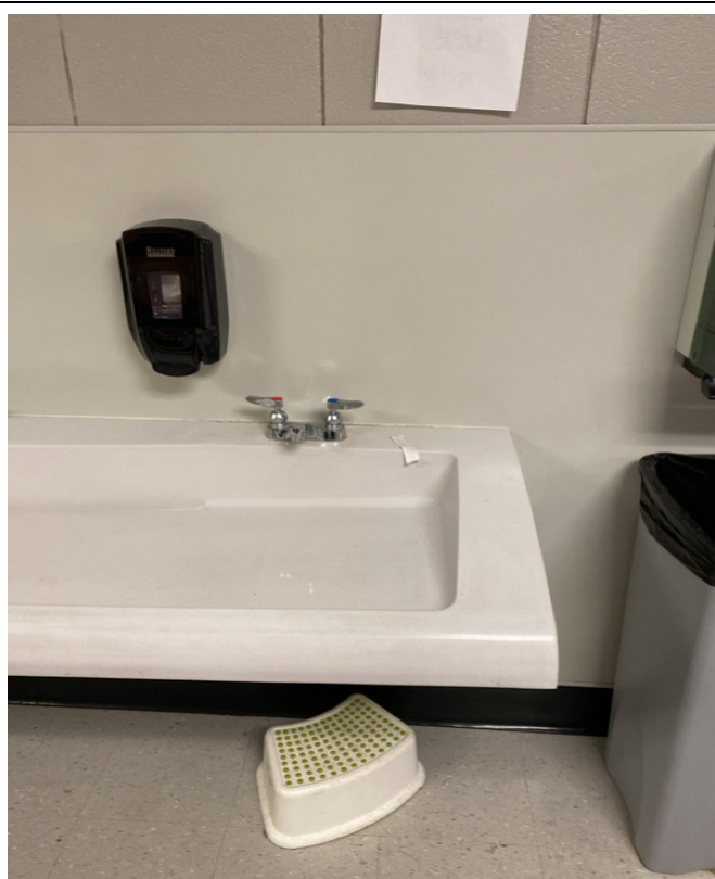
2/7/2024 - 304-16 - Primary School - East Hall by Office-Third from Left
